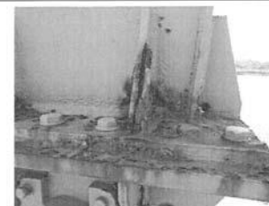
Inspection found heavy corrosion in the structure
