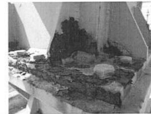
Inspection found heavy corrosion in the structure
